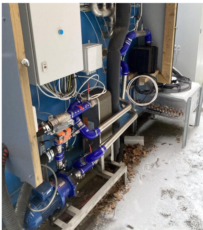
Figure 1. Coolant loop installations outside the container before addition of heaters and insulation. In the lower left corner, the Iwaki coolant pump is connected via piping to 3-way valve and Alfa Laval plate heat exchanger. The tubes going over the heat exchanger are connected to the fuel cell system inside the container. The black tubes the most left are the tubes connected to the Hydac cooler. On the right is the Ecocoil cooler for the component cooling loop.
